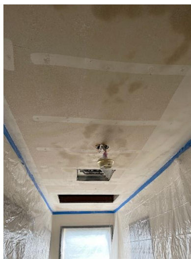
Hallway popcorn scraped off ceiling, texture applied, painted and new light.
