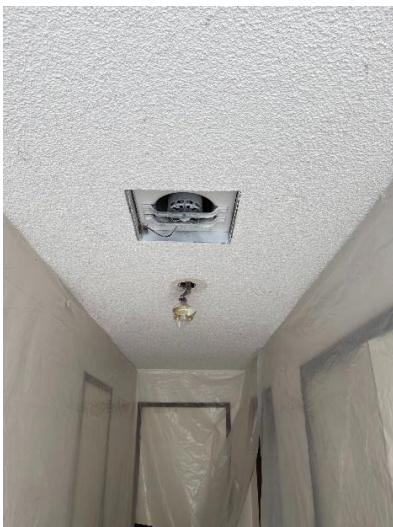
Hallway popcorn scraped off ceiling, texture applied, painted and new light.
