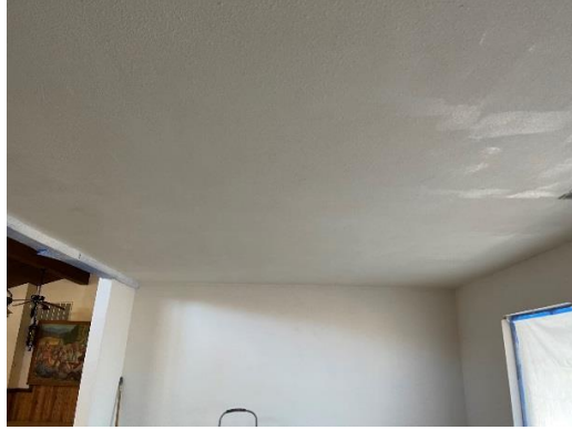
Primer painted on ceiling and walls
