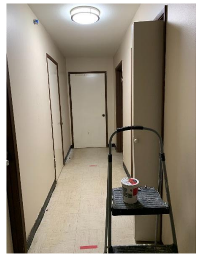
Hallway popcorn scraped off ceiling, texture applied, painted and new light.
